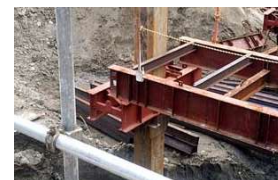
Downtown with top-down construction
